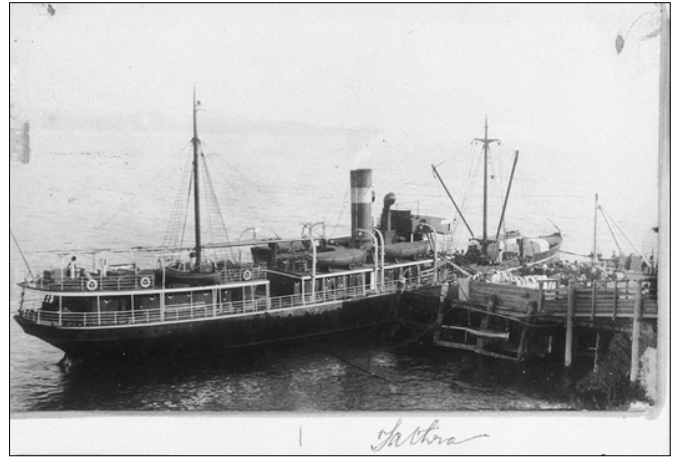
The ' Merimbula ' at Tathra Wharf. Photograph: State Library of NSW FL1698203
