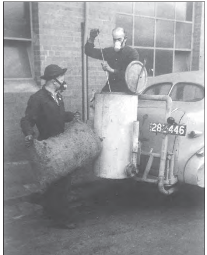
Hard Times: Cars were converted so they could be powered by a charcoal burner during WWII, when petrol was scarce. Photo: Australian War Memorial.
