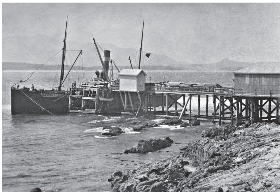
Loading timber at Bermagui wharf
