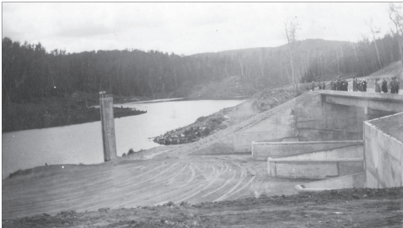
Cochrane Dam, presumably at its opening in 1958. Image courtesy Bega Valley Historical Society.
