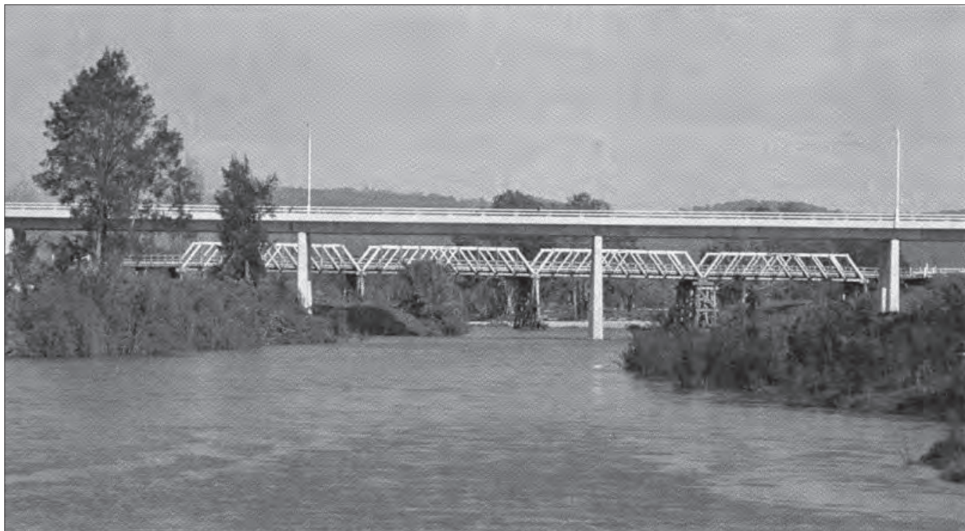
The old and new bridges, looking east along the Bega River, in 1975. At the time of construction, the new 624-metre long reinforced and prestressed concrete bridge was the sixth longest road bridge in NSW.
