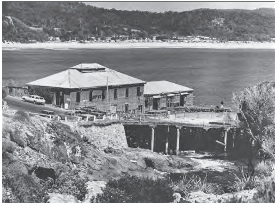
Tathra Wharf showing extent of deterioration c. 1970. The 1918 single-story shed was later demolished.
