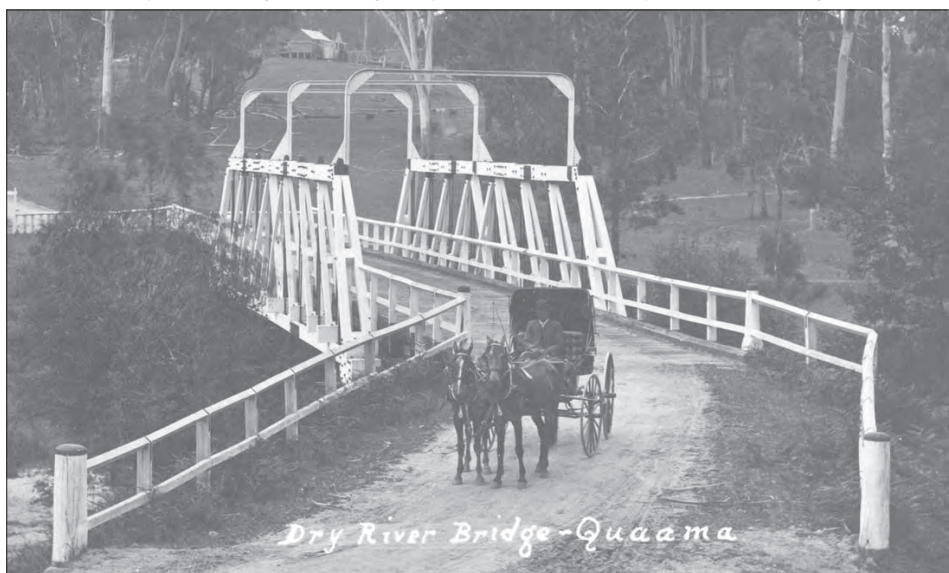
Time-travelling back to when the highway south included this Allan Timber Truss Bridge crossing at Dry River, Quaama
