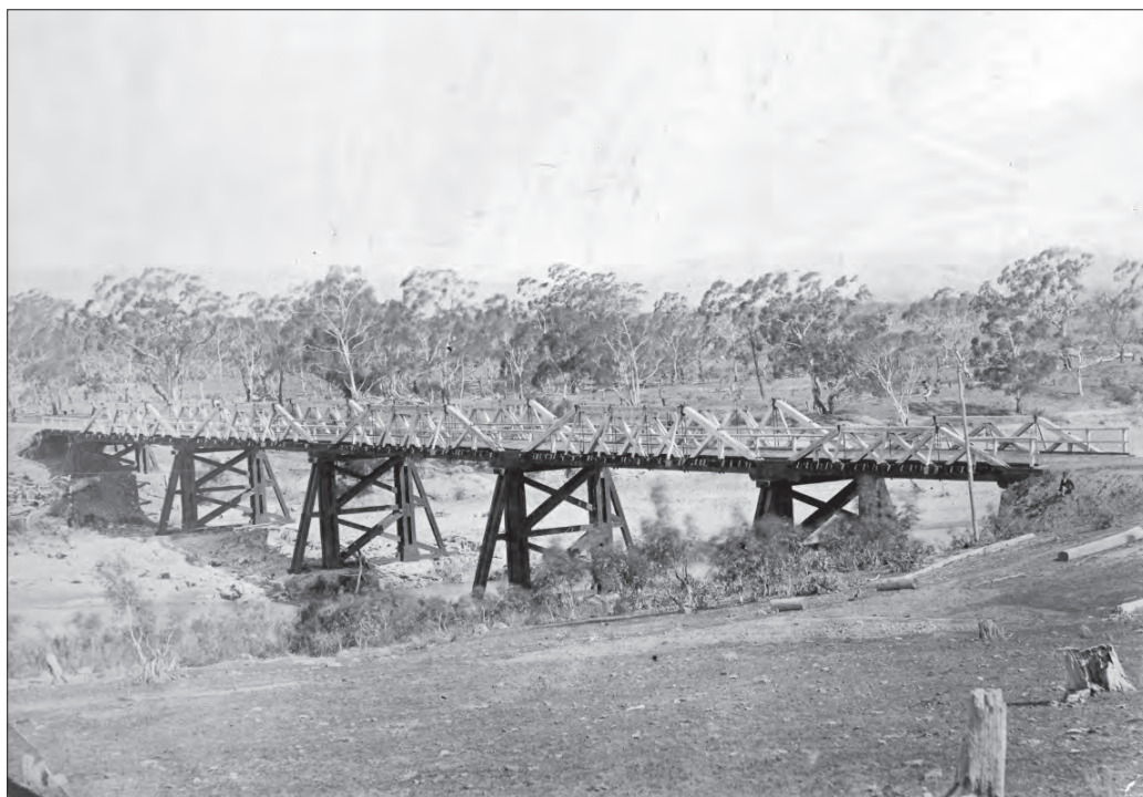
The timber truss Warri bridge
