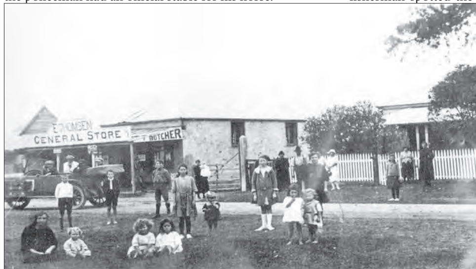
Guy’s Store and neighbouring residence were originally built in timber in 1869. In 1877 they were upgraded with convict made bricks that came to Batemans Bay as ship’s ballast. By the 1920s Guy’s Store was trading as Thomsen’s Store.
