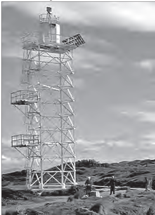
The 15 metre tall metal skeletal tower at Green Cape that was commissioned in 1992.
