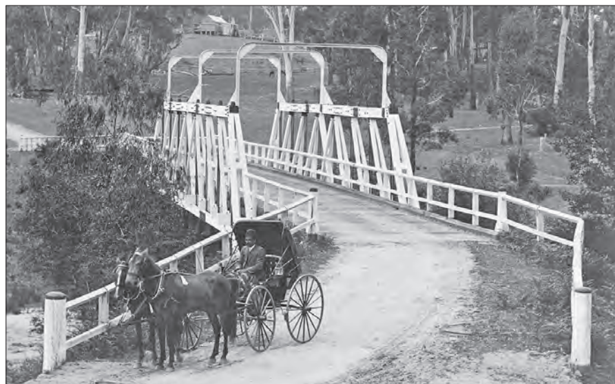
The bridge over Dry River at Quaama, c 1912.
