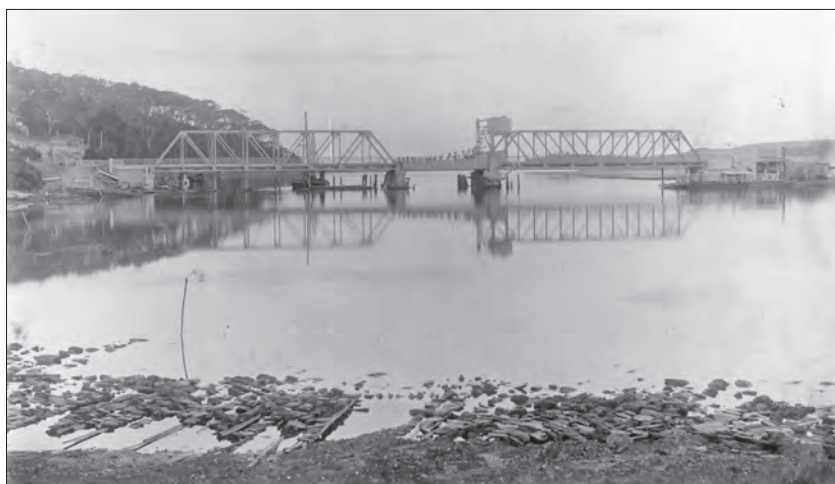
The Narooma bascule span bridge
