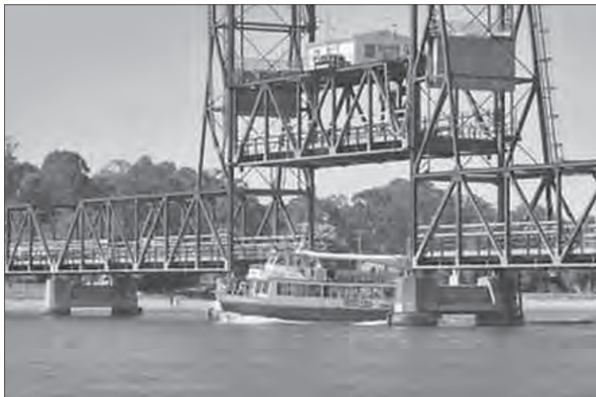
The old Clyde River Bridge at Batemans Bay. This opened to traffic in November 1956 and was replaced by the current bridge in February 2023.
