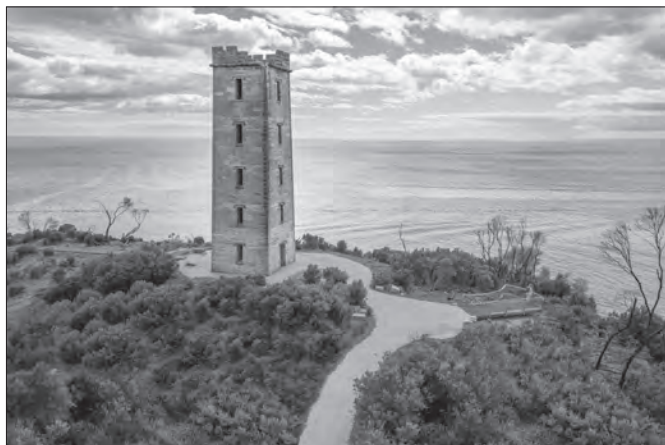
Boyd's Tower, Twofold Bay
