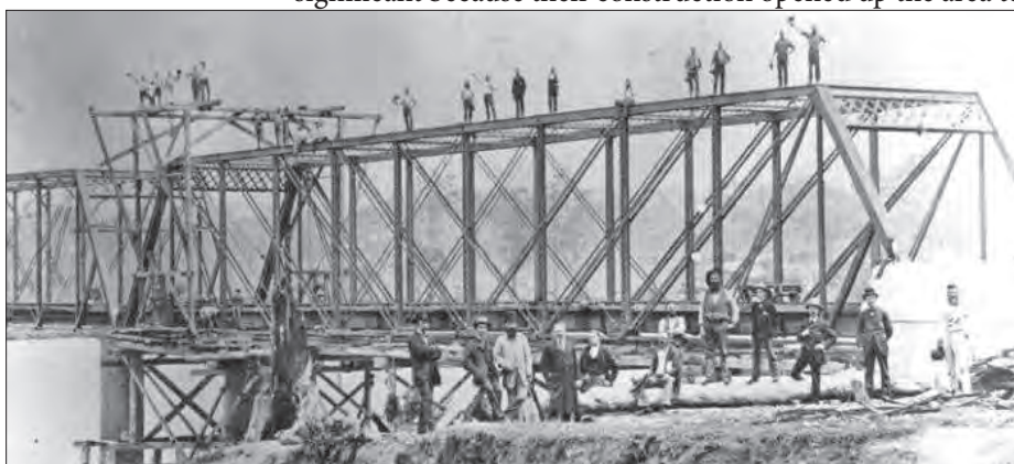
Construction of the old Shoalhaven Bridge at Nowra
