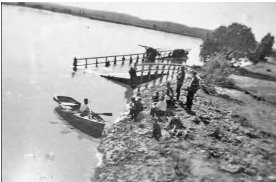
The Moruya Bridge after the 1945 flood
