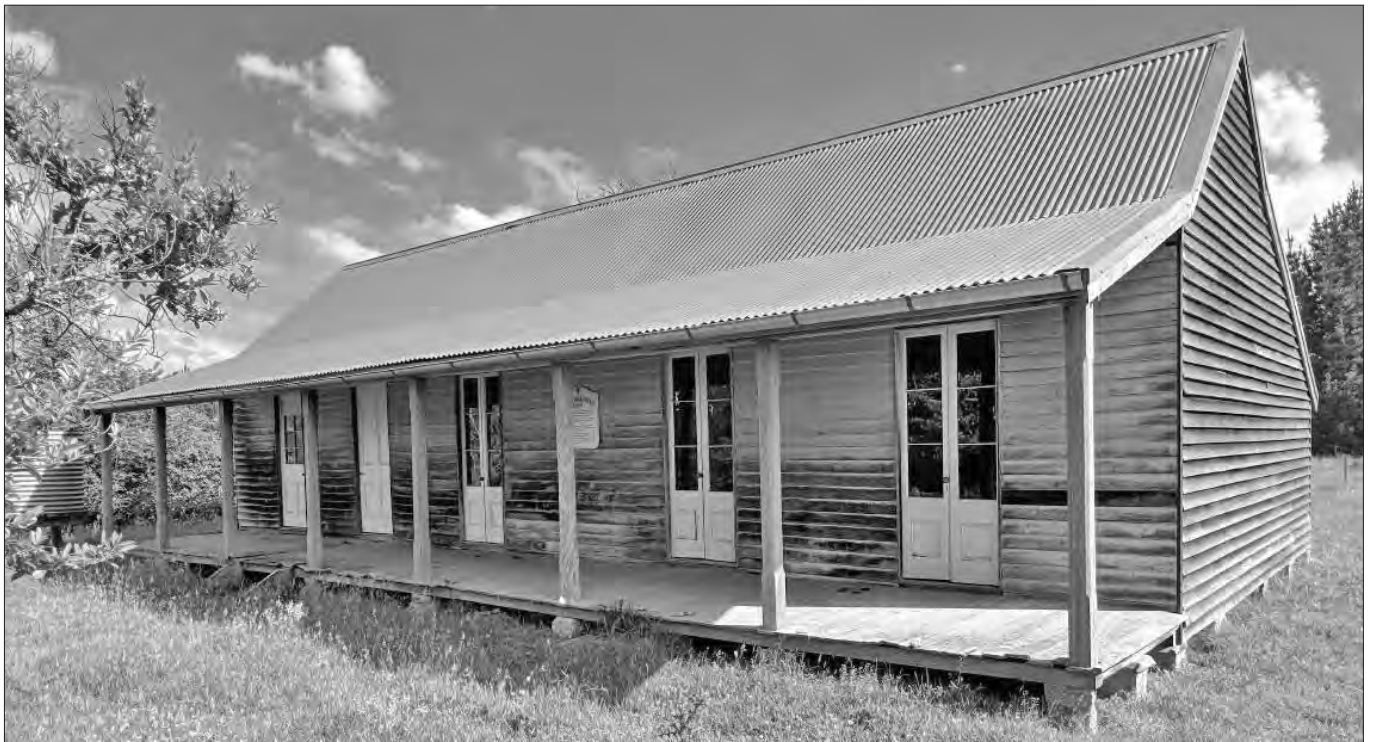
The building was lovingly restored in 2001. Picture by Tim the Yowie Man.
