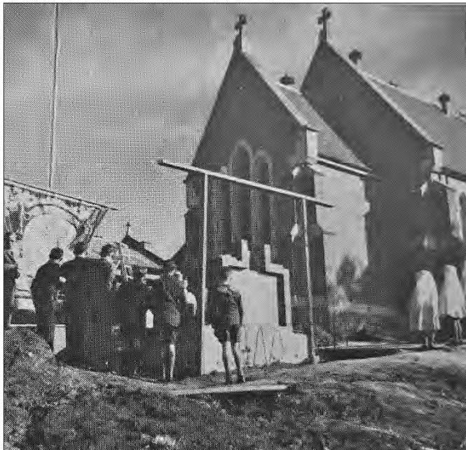
A newspaper photograph from the laying of the foundation stone at St Patrick's Bega, in 1951
