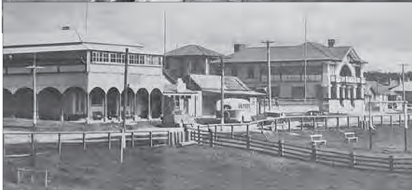
Top: An aerial photo of Bermagui from 1937 when Bermagui had a steamer wharf. The Beach House was prominent. Above: The building was renovated and altered in the 1940s and 1950s. Arches were added at the front and side and the verandah was enclosed on the top level. (Our thanks to Bermagui Historical Society for assistance in providing the above information.)
