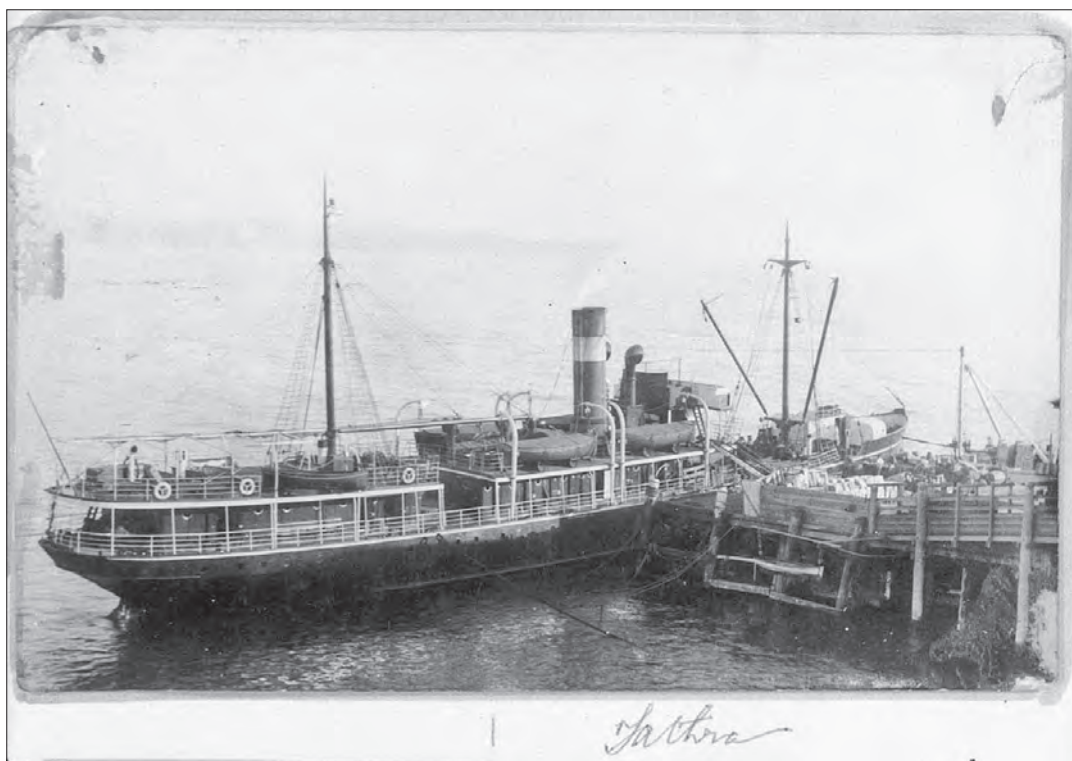
The 'Merimbula' at Tathra Wharf. Photograph: State Library of NSW FL1698203
