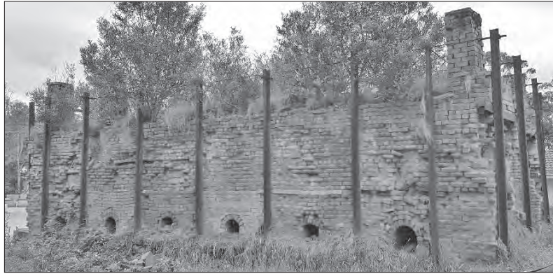
The first of the down-draught kilns constructed at Kalaru.
