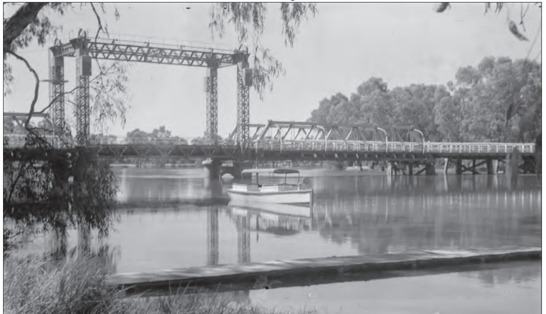
The Allan Timber Truss Bridge over the Murray River at Swan Hill, this is the oldest remaining timber truss lift bridge in NSW. Image State Library of Victoria, 10381/64608
