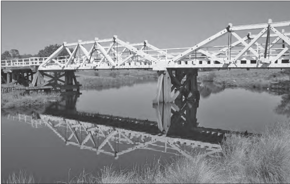
Crankies Plain McDonald Truss Bridge near Bombala
