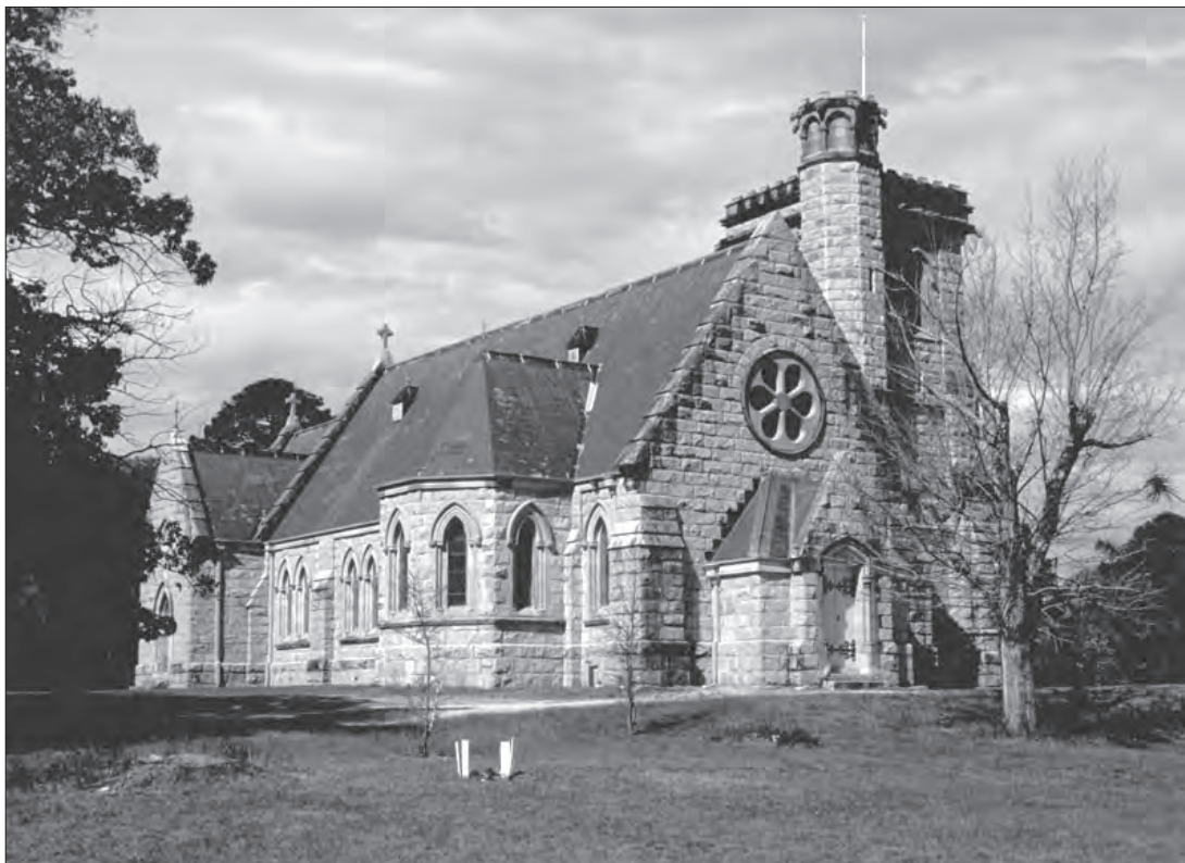
All Saints Anglican Church, Bodalla. Thomas Mort was a prominent Anglican layman. He and his first wife, Theresa, chose the site and had plans drawn up by noted Sydney architect Edmund Blacket. Mort also ordered windows from England. When Mort died in 1878, Bodalla residents decided to erect a memorial window in the church so, at the family’s request, Blacket enlarged his original plan for the church and included a rose window on the west end. The church was completed in 1901 and is a memorial to Thomas and Theresa.
