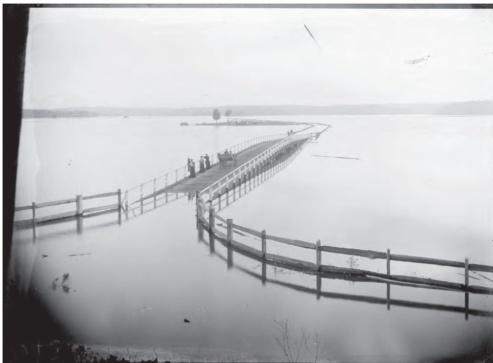
Two views of Wallaga Lake Bridge — under construction and under flood, c. 1894 to c. 1900. (see story page 15) Images: From 'Negatives of Glass', courtesy Bermagui Historical Society, and National Library of Australia, nla.obj-1403341238-1
