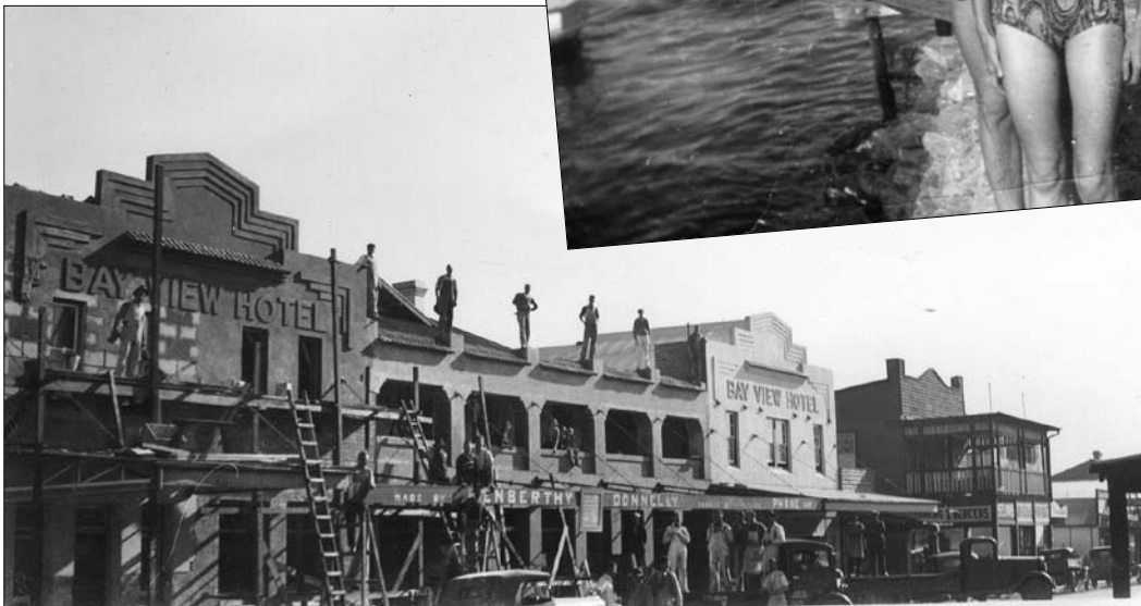
Bayview Hotel being renovated, 1940s.
