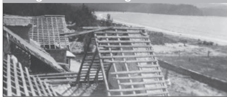
Below: After removal of weather-damaged roof framing.
