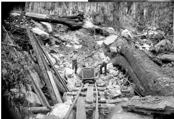
Hydraulic Sluicing up Tilba Creek in 1899. Sluicing yielded some gold from areas previously worked by prospectors but caused massive environmental damage.
