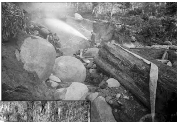
Hydraulic Sluicing up Tilba Creek in 1899. Sluicing yielded some gold from areas previously worked by prospectors but caused massive environmental damage.
