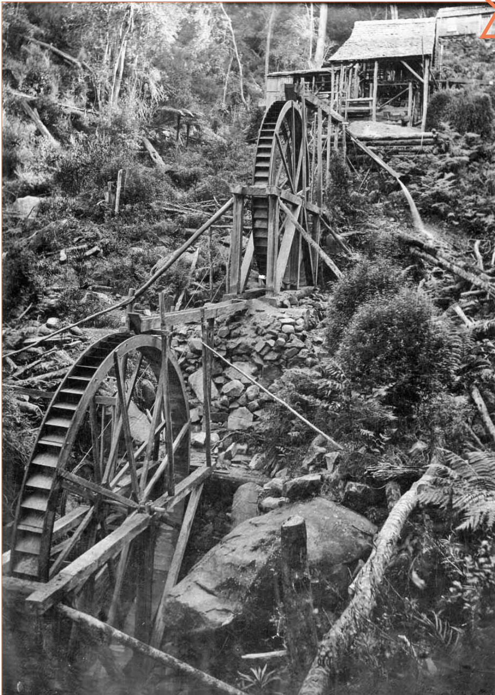
Water wheels used for generating power to drive a small stamper battery on Mount Dromedary in 1910. William Robert Easdown photographic collection, National Library of Australia. See story pages 12 to 15.
