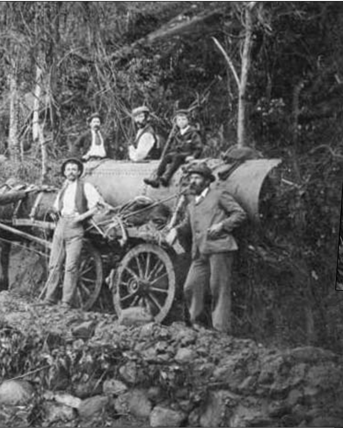
Men hauling boiler to Mt Dromedary Mine, 1900. Richard Mossop Bate. Block and tackle were often used to haul heavy loads on mountain tracks. Image from William Robert Easdown
