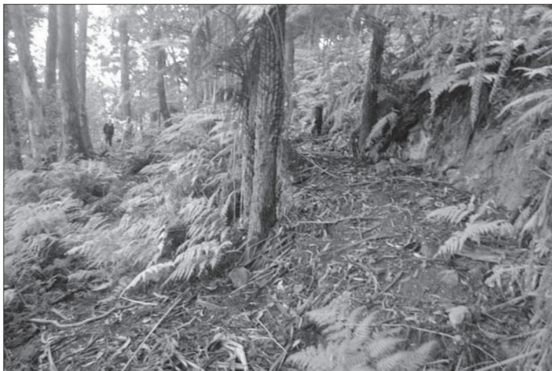
The Shoebridge Track had significant traffic and in several locations short lengths of 'passing lanes' were constructed. Here the passing lane is on the right and rejoins the main track where the man is standing. Photo: www.accessforall.asn.au
