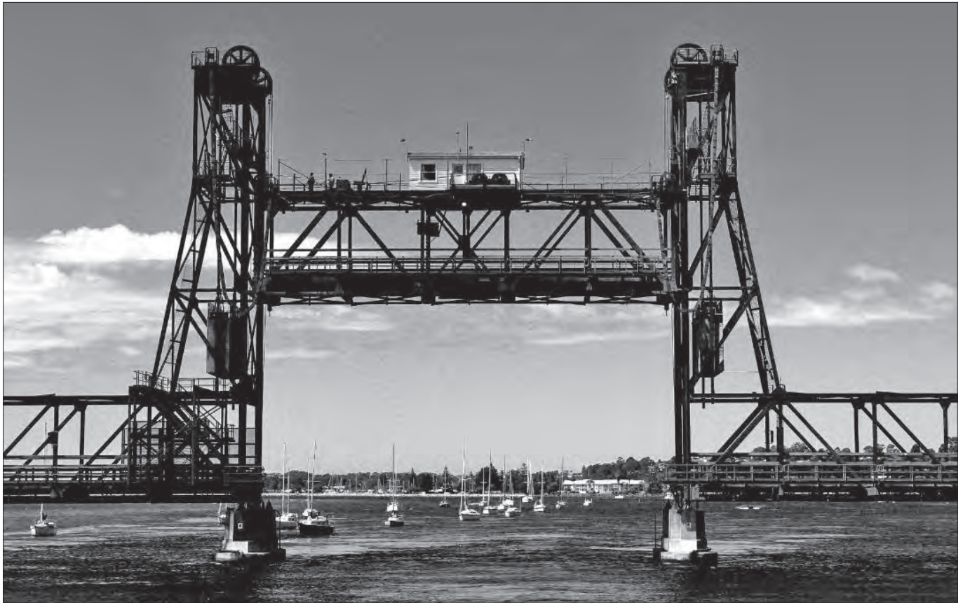
Batemans Bay Bridge Raised...Counterweights Dropped. Note Bridge Operator standing to left of control house. Photograph by Ted Richards.
